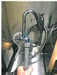
2 JUC FILLER FAUCET COORDINATE WITH PLUMBING DRAWINGS
