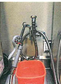
1 JUC FILLER FAUCET COORDINATE WITH PLUMBING DRAWINGS
