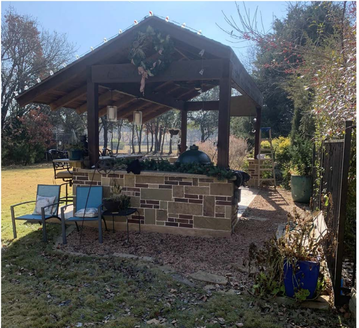
Remodeled Roofline to Clear Easement
