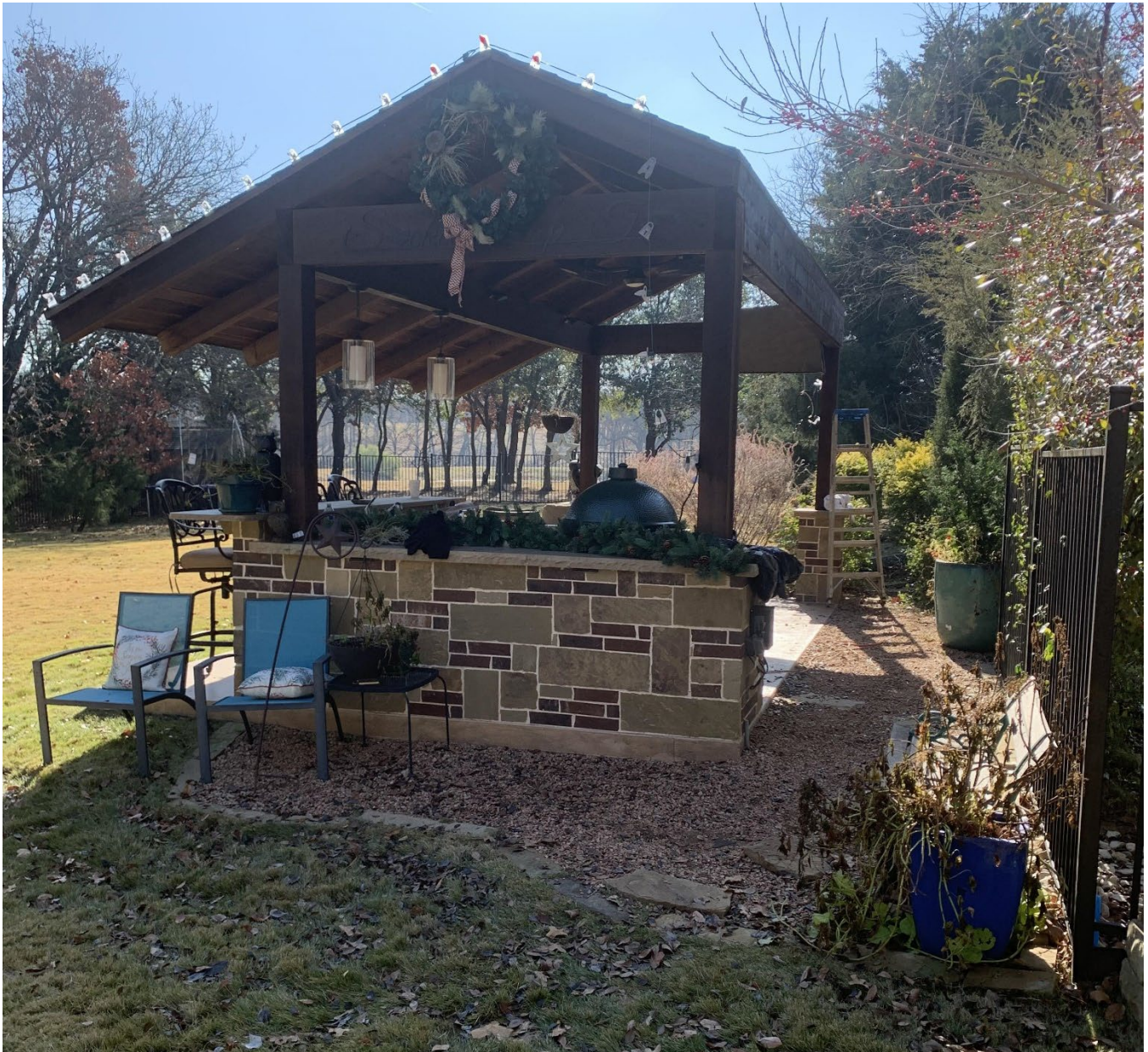
Remodeled Roofline to Clear Easement
