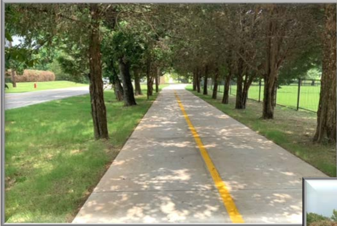
John McCain Road Trail and Misc. Sidewalk Connections Contract Amount $935,249.50
